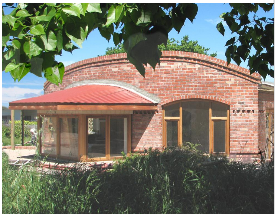
Newly completed Phase 2 of Timour Hall Cottages. Photo by Malcolm Attfield.
