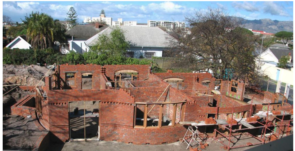
Building Progress as on 22 nd July 2012. Photo by Malcolm Attfield.
